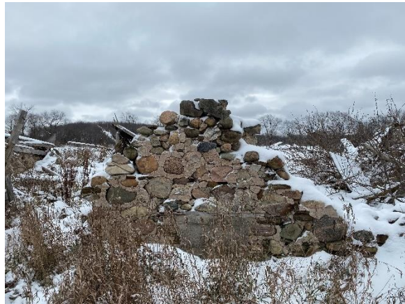
Plate 28: Parged fieldstone walls of Structural Foundation No. 2
