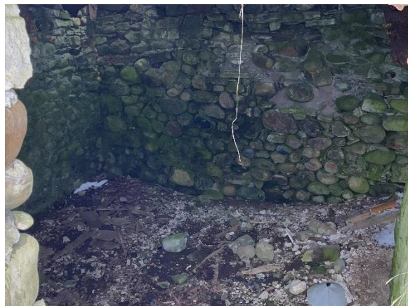
Plate 32: Fieldstone wall of below grade cellar interior
