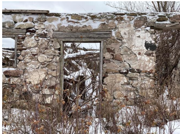
Plate 21: Parged fieldstone wall and doorway
